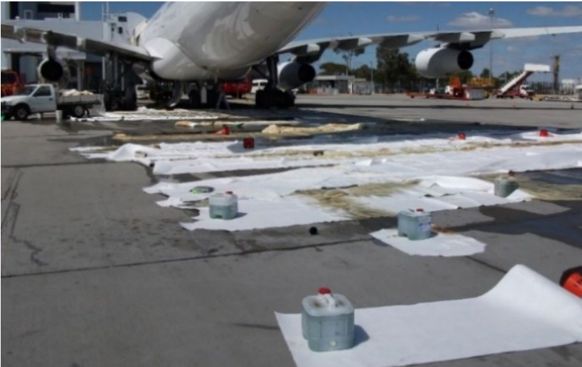
Substantial & Hazardous Fuel Spill
