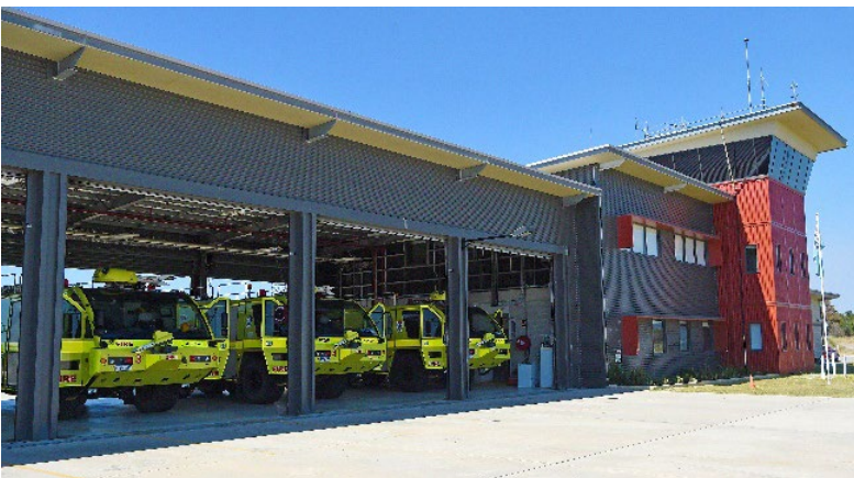
Aviation Rescue Fire Fighting Services (ARFFS) Station Perth Airport
