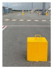
Concrete tie-down blocks are designed and engineered to withstand the harsh weather conditions and withstand the dangerous uplift of high wind speeds.
