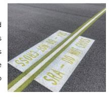
Where possible, the SRA is fenced around the manoeuvring area which is monitored by radar and includes signage. Where fencing is not possible, the SRA is bound by a continuous double green line highlighted white in the centre.
