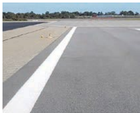
Runway edge markings
