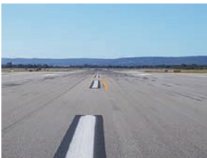
Centreline runway markings
